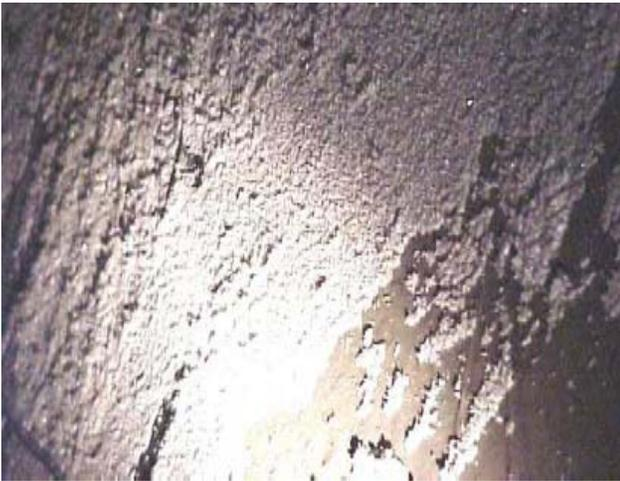
Figure 13. HDC Tower – Scale on Sidewall
