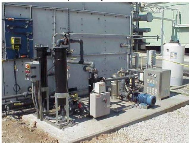
A 20 gpm unit was sized and selected by the supplier for Mt. Holly. HDC units are sized to treat the entire system volume seven times a day plus an allowance for makeup water. Based on the size of this tower and expected heat load this would have calculated to a 15 gpm unit, but the HDC supplier elected to increase to the next larger size in their product line, a 20 gpm unit, rather than use their smallest 10 gpm model.
