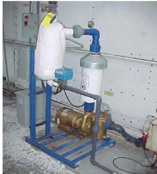
The PP supplier prefers to size their units to turn over the system volume once every 15 minutes for good microbiological control. The initial 110 gpm flow rate through the 3 in. unit created a 10-minute turnover frequency. When a larger 6-inch unit was installed, the turnover frequency increased to once every 2 minutes.
